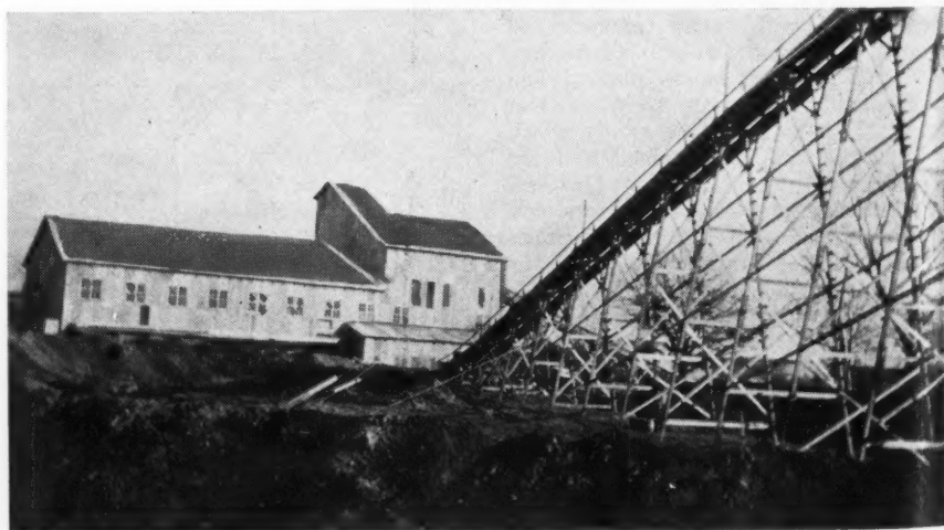
NEW SHORT CREEK MILL of Tri-State Zinc Co., near Galena, Kan., which is designed to re-treat 50 tons per hour of mill tailings excavated from the creek bed. Between 500,000 and 600,000 tons of tailings, the accumulation of decades, is available. The mill uses screens, rolls, and tables. Victor C. Allen, of Joplin, is general superintendent
